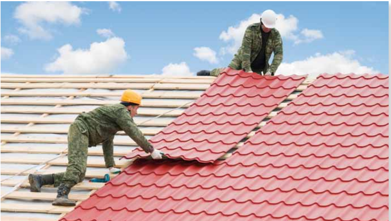
Installing a steel roof.
