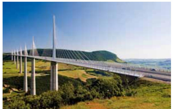
Millau Viaduct (France)
