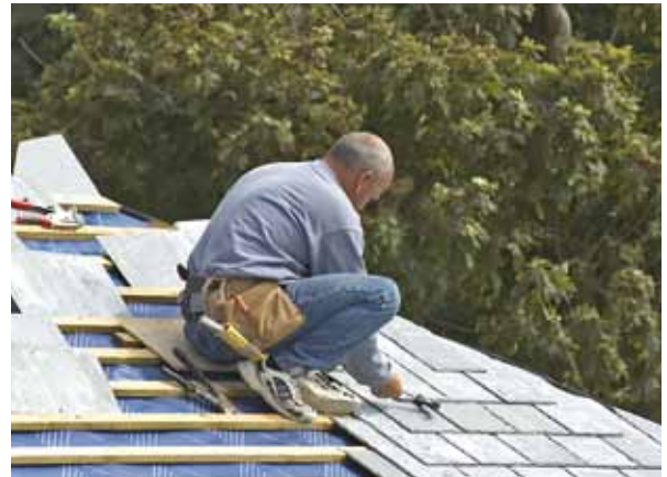
Laying of slate roofing tiles.
