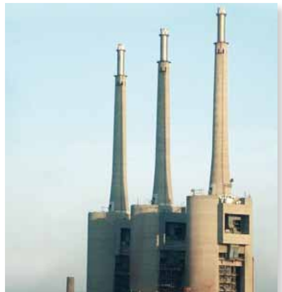
Conventional power plant
